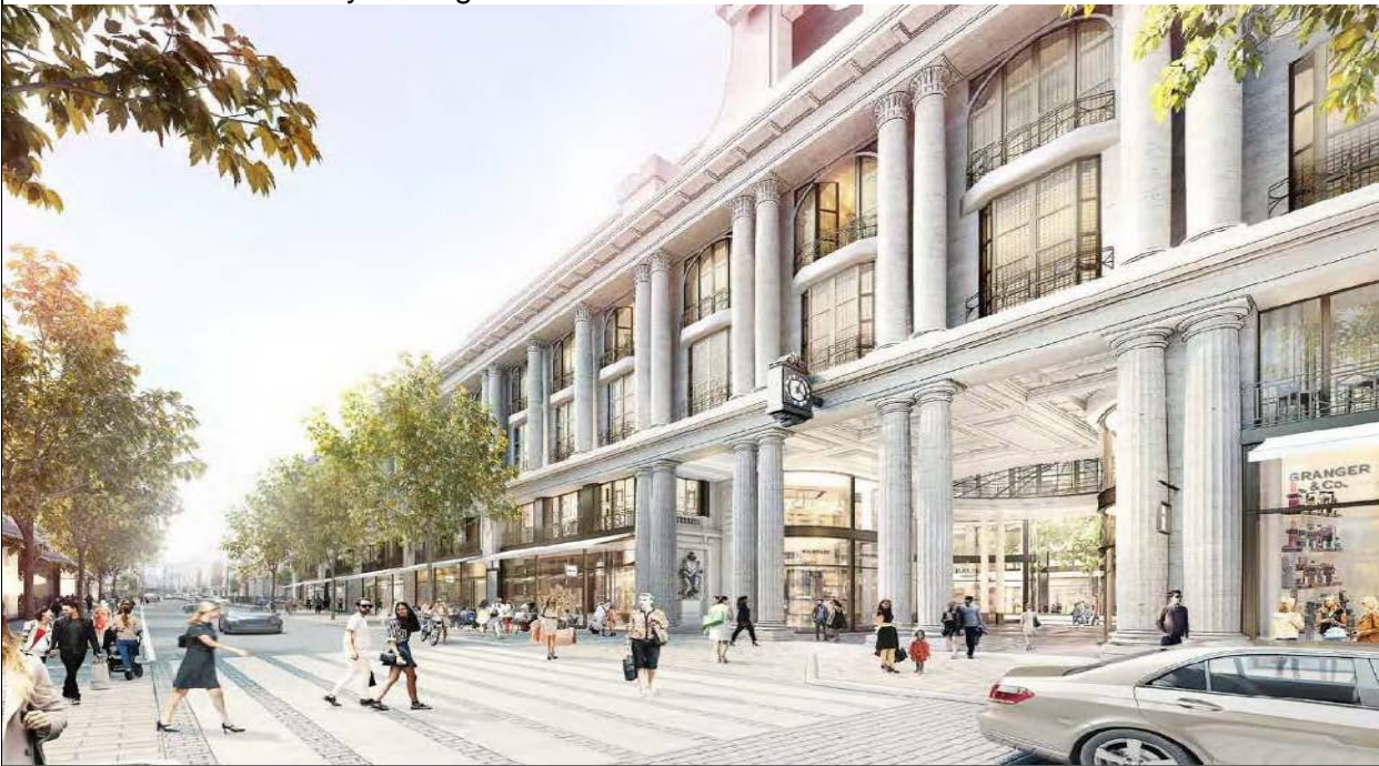
Visual of the Queensway frontage
